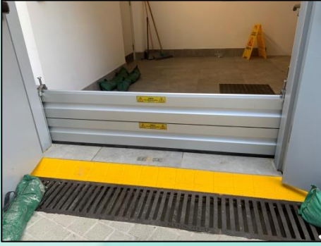
At entrance of staircase
