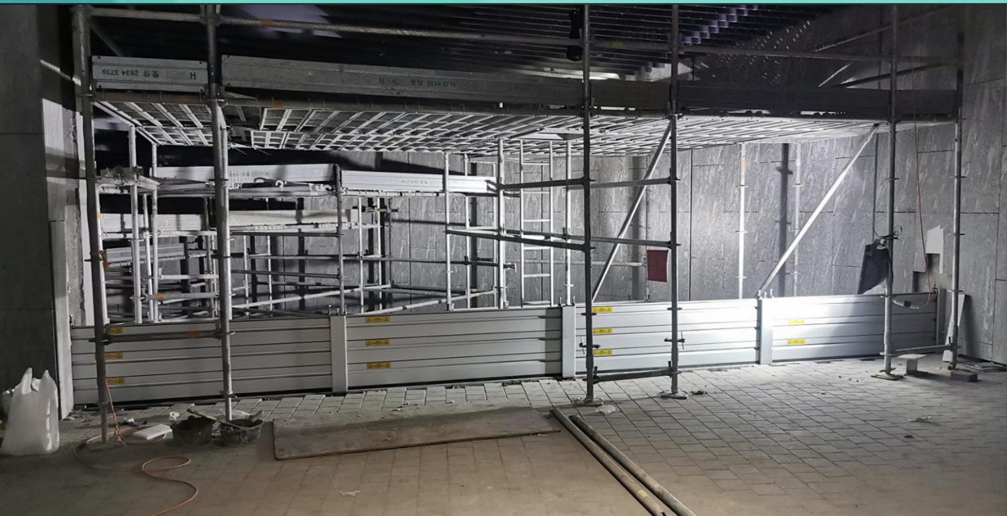
For wide car ramp ( under construction )
